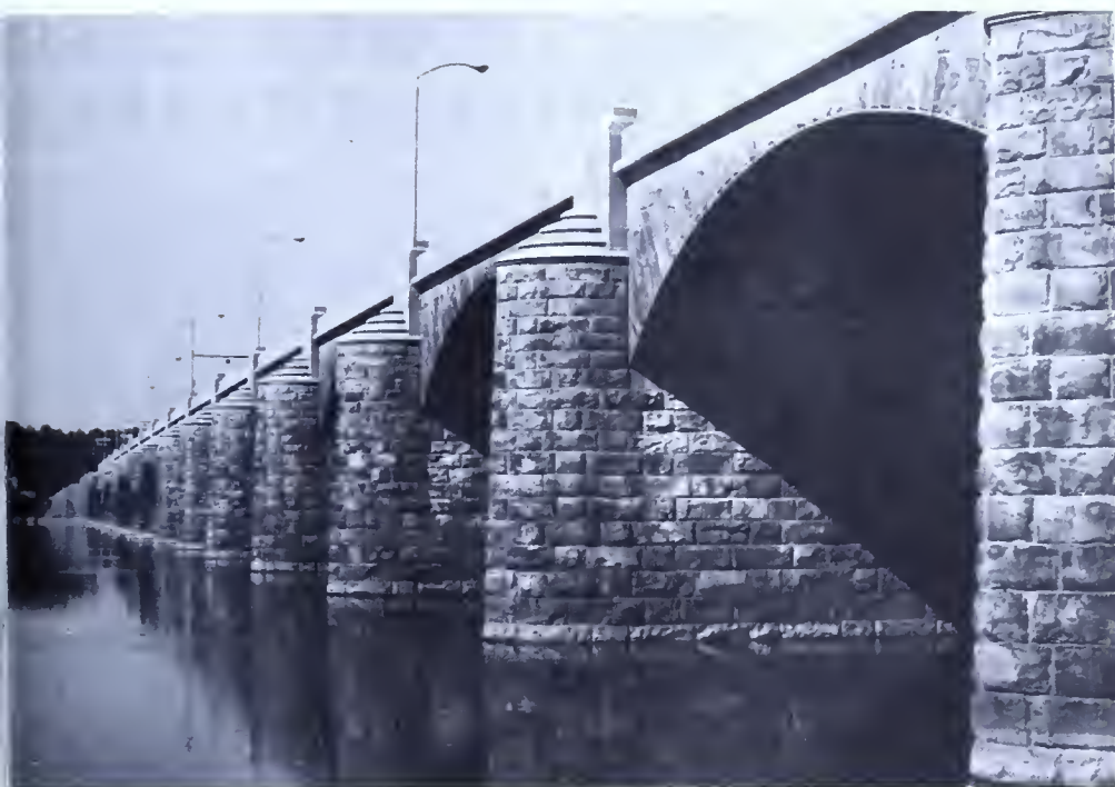
Market Street Bridge over the east channel of the Susquehanna River.
